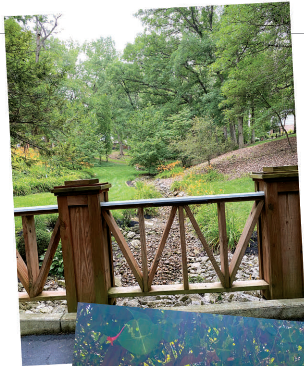
ABOVE: GARTLAND BRIDGE
