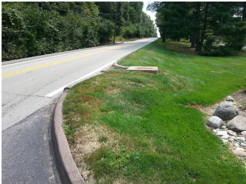
Figure 1-1. Photo of Current Stormwater Drainage System Near Twin Fawns Subdivision
