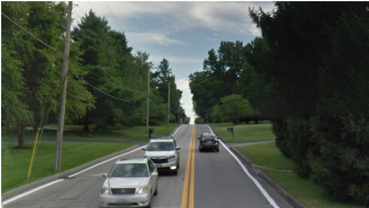
Geyer Road at Clayton Road – Looking South
