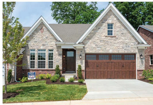
The Arbors at Frontenac
